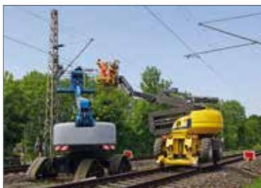
Construction of contact lines
