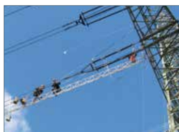
Overhead line construction
