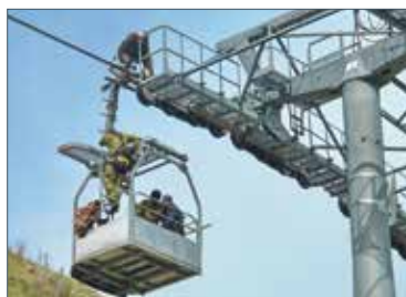
Cable car construction
